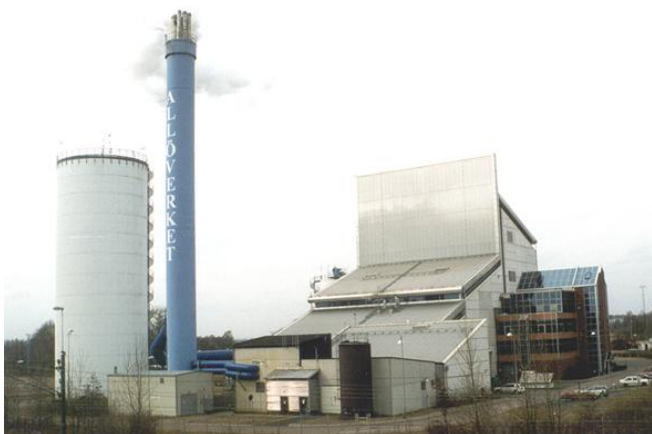
Allöverket, combined power and heating plant, fuelled by bio-mass.
