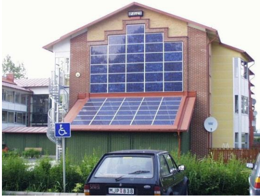
Solar panels in the residential area of Österäng.
